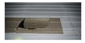
Photos. Top photo shows the panel where a fire fighter fell through a translucent corrugated roof panel. The panel was flush with the surrounding roof surface. Bottom photo shows an aerial view of the building where incident occurred. The translucent roof panels appear grey against the white metal roof. At night, the panels are difficult to detect and typically do not include a frame.
