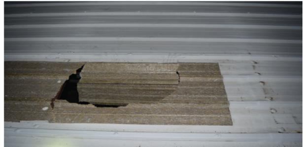
Photos. Top photo shows the panel where a fire fighter fell through a translucent corrugated roof panel. The panel was flush with the surrounding roof surface. Bottom photo shows an aerial view of the building where incident occurred. The translucent roof panels appear grey against the white metal roof. At night, the panels are difficult to detect and typically do not include a frame.
